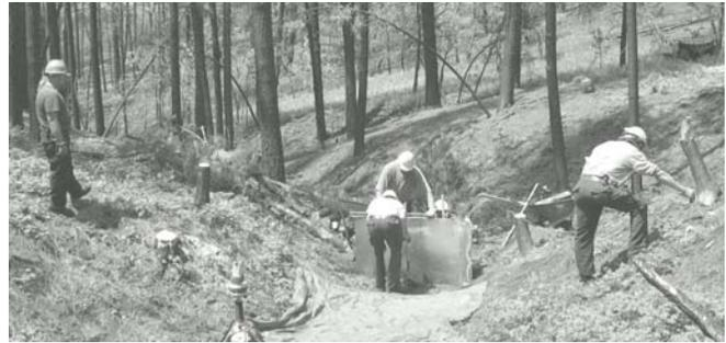
Figure 1. Sheet metal cut-off wall installation.
