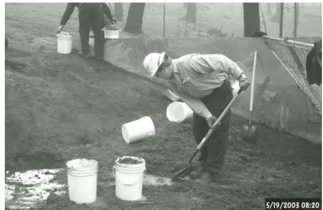
Figure 4. Buckets are used for sediment clean out.
