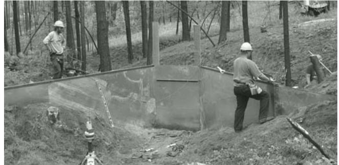
Figure 2. Sidewalls of sediment trap.
