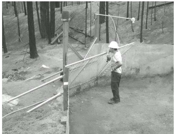
Figure 3. V-notch weir and trash/debris screen.
