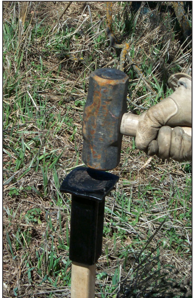
Figure D1 —Steel cap for pounding wooden stakes into the ground.
