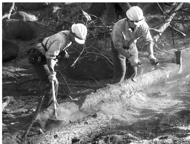
Fig. 7. Fire crews install a contour-felled log erosion barrier in a research catchment after the 1999 Mixing Fire (California, USA).
