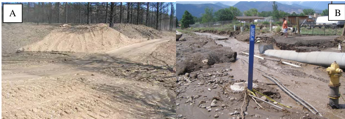
Figure 2. An example of (A) successful culvert removal and construction of low-water crossings on National Forest lands; and (B) a bypassed and breached, undersized culvert on private property, Schultz Fire, Arizona.
