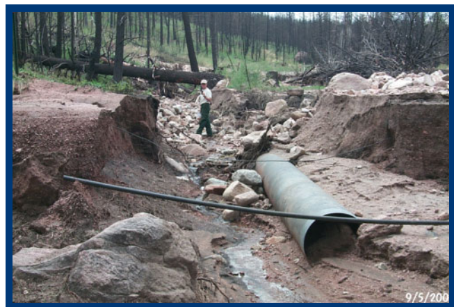
Figure 10.11 —Rocky Mountain Research Station Engineer Joe Wagenbrenner surveys a channel scour, following the Hayman Fire, 2002, Pike-San Isabel National Forest near Deckers, CO. (Photo by A. Covert).
