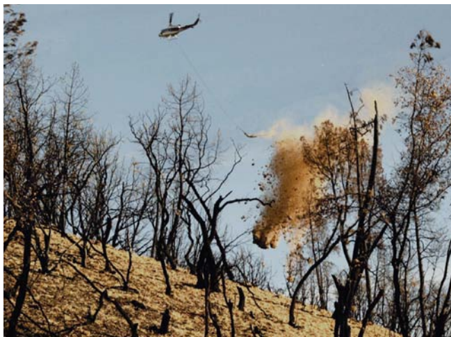
An aerial application of straw mulch treatment is released over the target area by a cargo net suspended below a helicopter. (photo from Burned Area Emergency Response Treatments Catalog by C. Napper (2006); p. 25)
