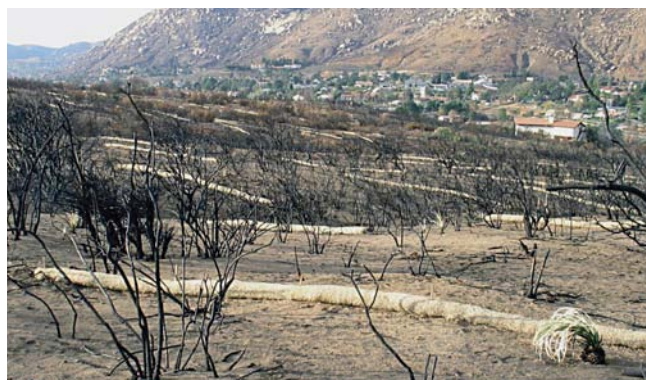
On a burned hillslope in southern California, straw wattles were installed in a staggered layout.
