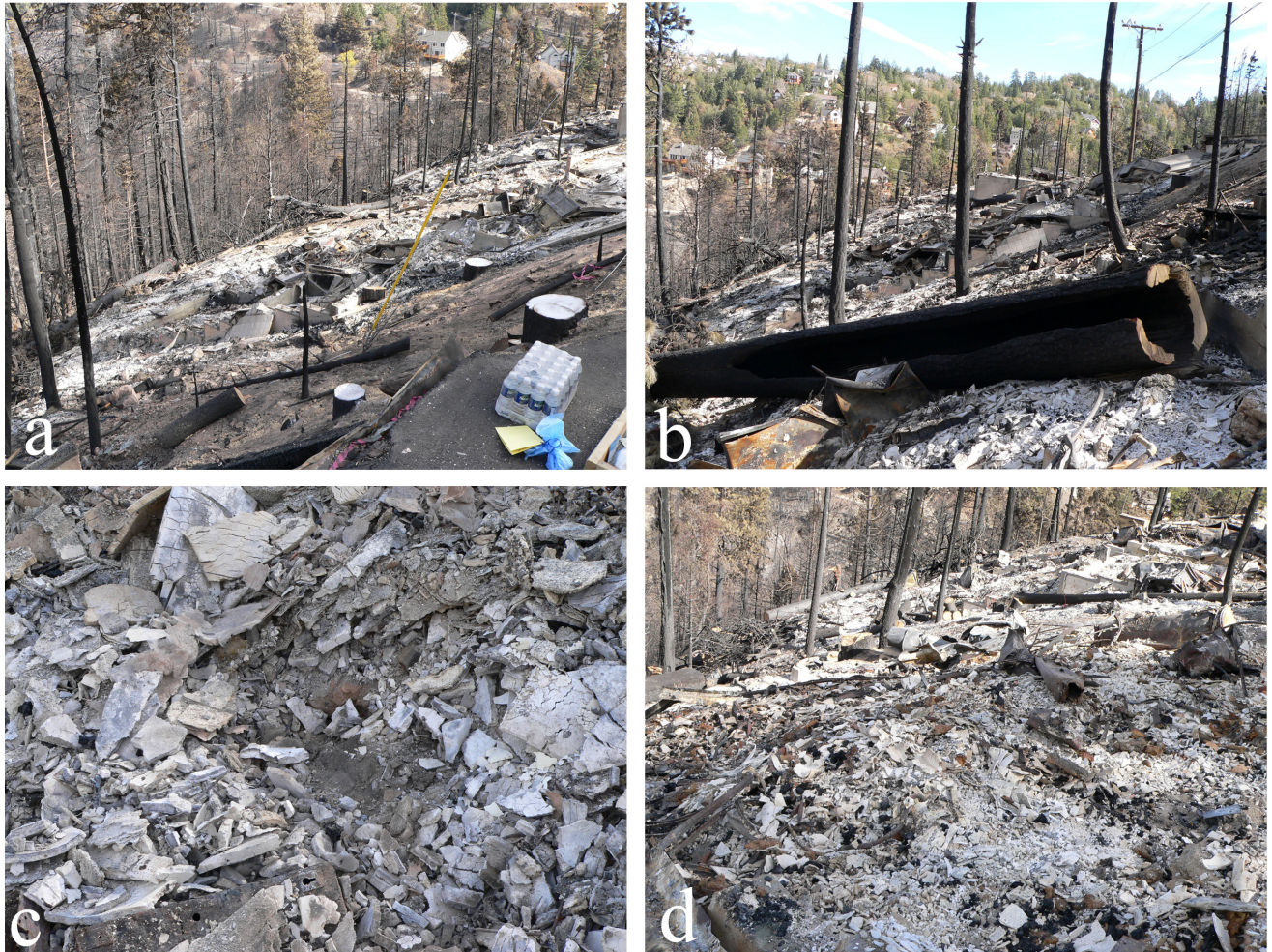
Figure 40. Photographs of some of the burned structures sampled at the GrassValley01 location.
