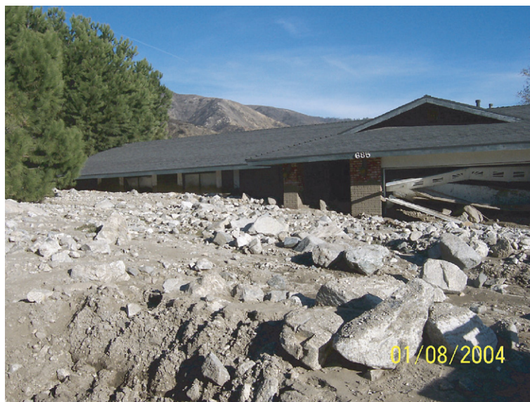
Fig. 1. Photograph of a home buried by debris flows in Devore, California on Dec. 25, 2003.
