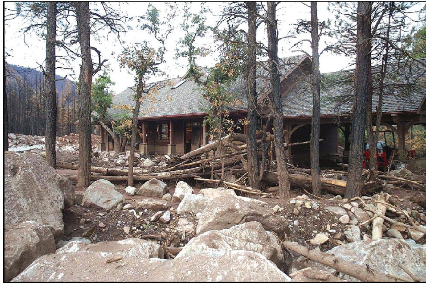
Fig. 9.2 House damaged by debris flow generated from 2002 Missionary Ridge Fire in southwest Colorado (USA)
