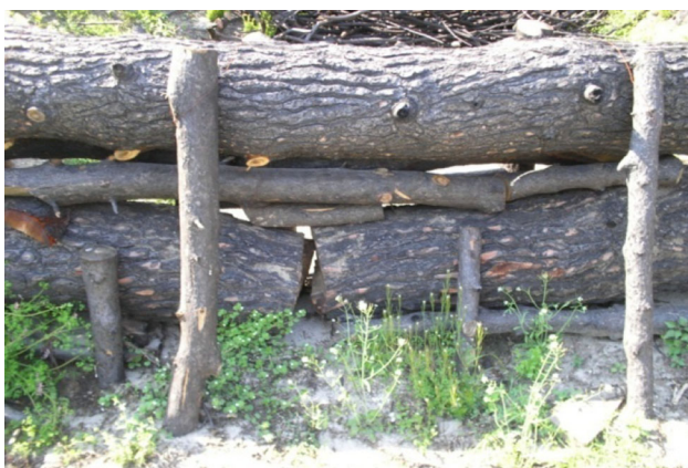
Fig. 7 Gaps between the logs of the log-dams and the resultant absence of sediments
